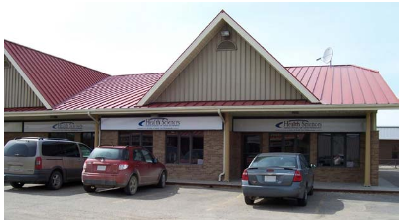
The new office at #12 - 395 Park Street
